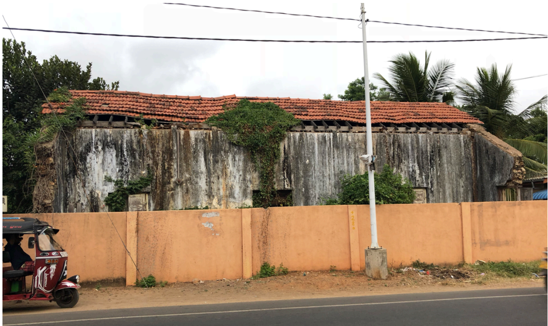
Photo 5. Road widening and destruction of traditional housing
