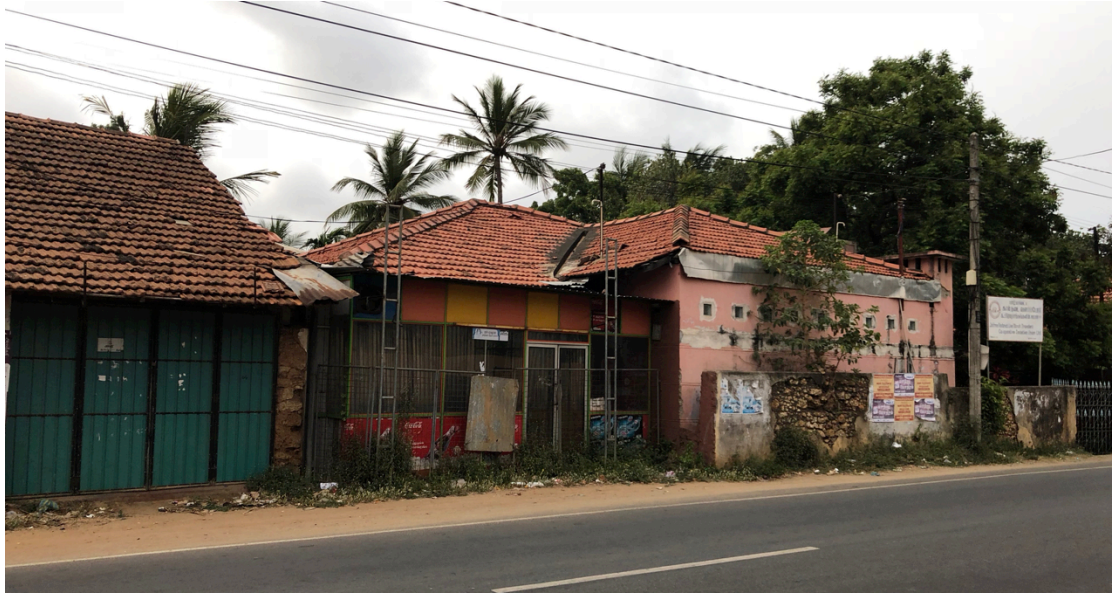
Photo 4. Road widening and destruction of traditional housing
