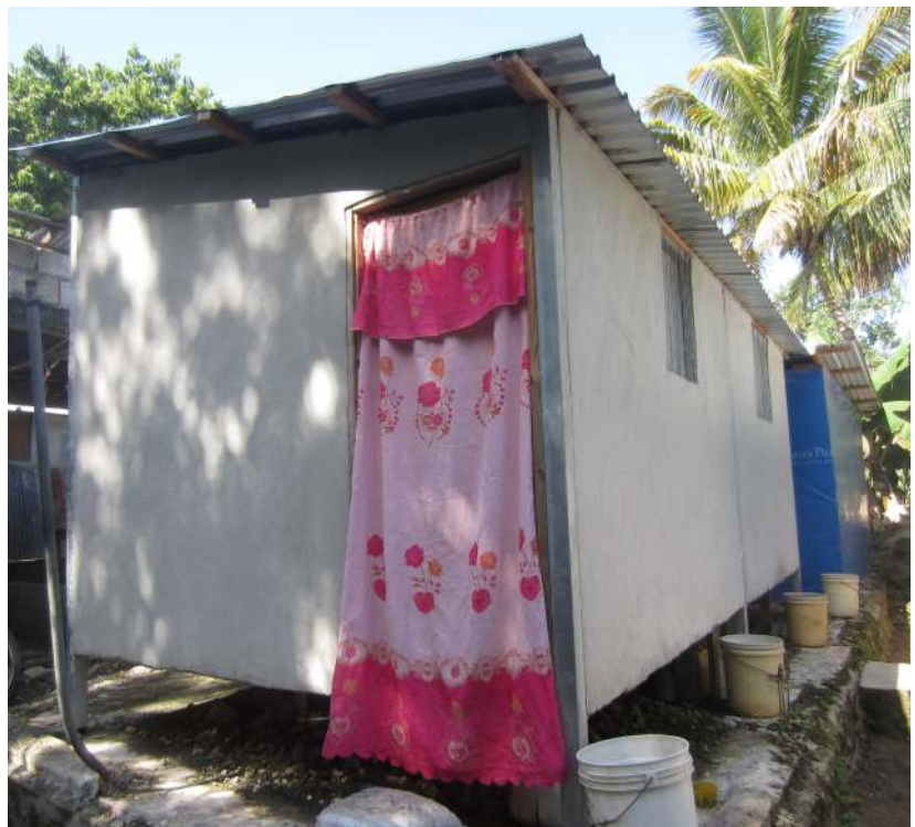
Figure 10: NGO-C, t-shelter C5
