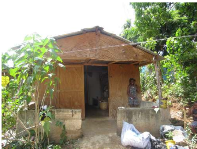
Figure 16: Example of repaired home (t-shelter A7)
