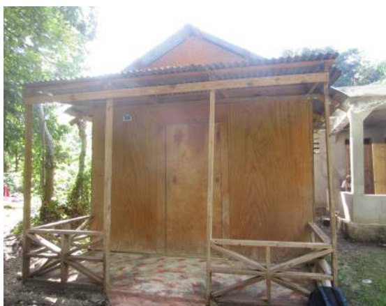
Figure 13: Color added to the concrete slab foundation (t-shelter A3)
