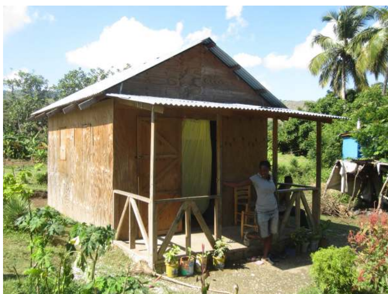
Figure 11: NGO-A, t-shelter A2
