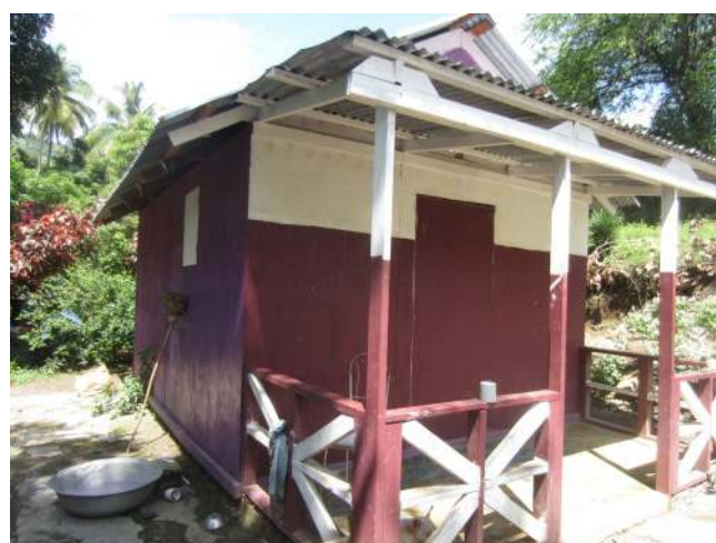
Figure 15: Painted t-shelter (t-shelter A7)
