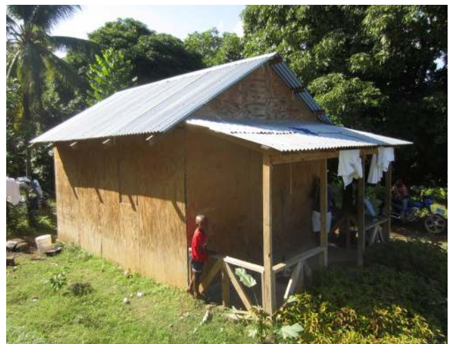
Figure 7: NGO-A t-shelter A1
