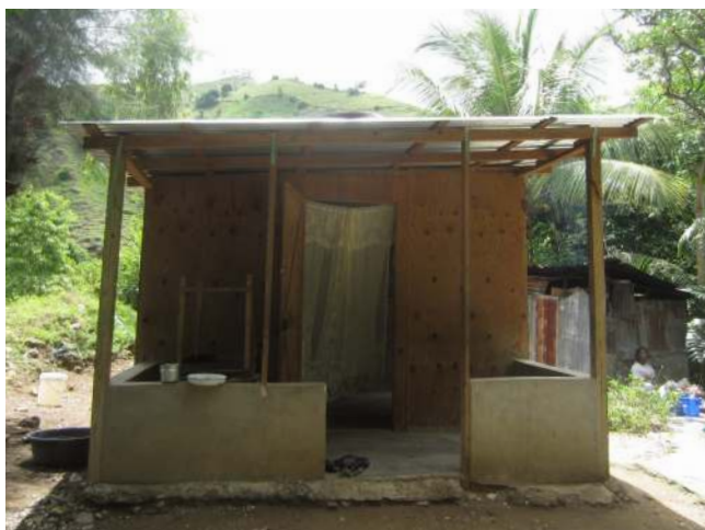
Figure 14: Concrete fenced porch (t-shelter A9)
