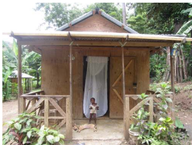
Figure 20: NGO-A t-shelter A29
