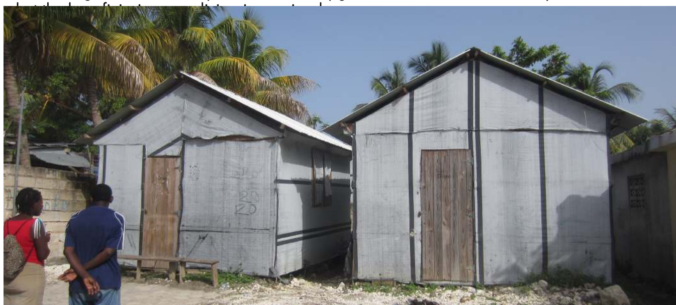
Figure 25: Abandoned t-shelters (B25 and B26)
