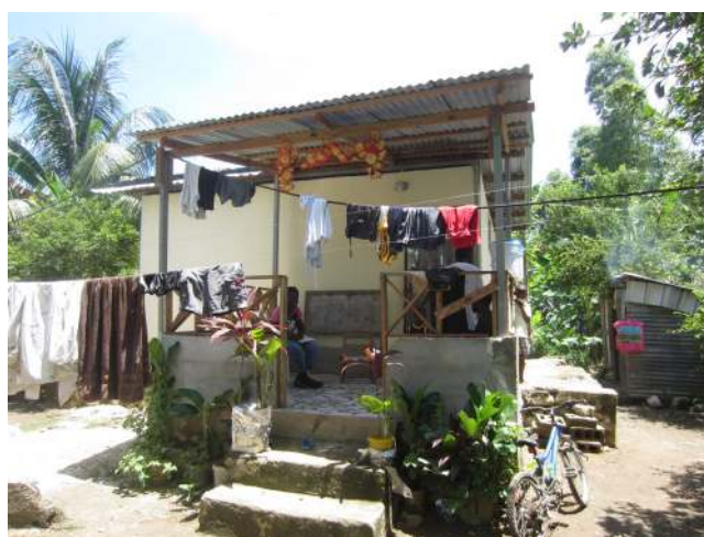
Figure 30: Steel polls recycled from a t-shelter sold for parts (t-shelters C16 and C17)
