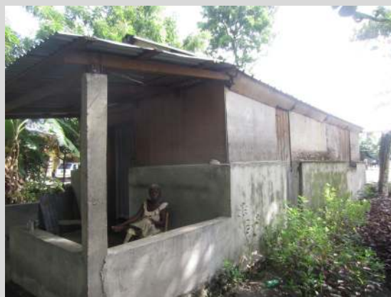
Two t-shelters (B27) put together to make one
