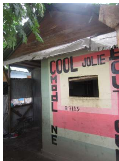
Figure 22: Business built onto t-shelter (B11)
