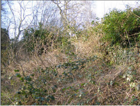
Figure 4.5: Overwhelming vegetation in the un-restored sections. The wall is to the right in the photograph (Source: author).
